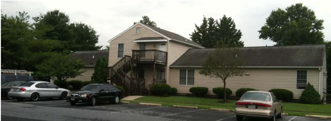
Existing Building Façade
